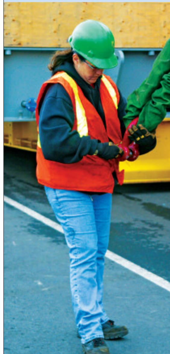
A longshore worker places a shackle on a sling in preparation for a heavy lift.
