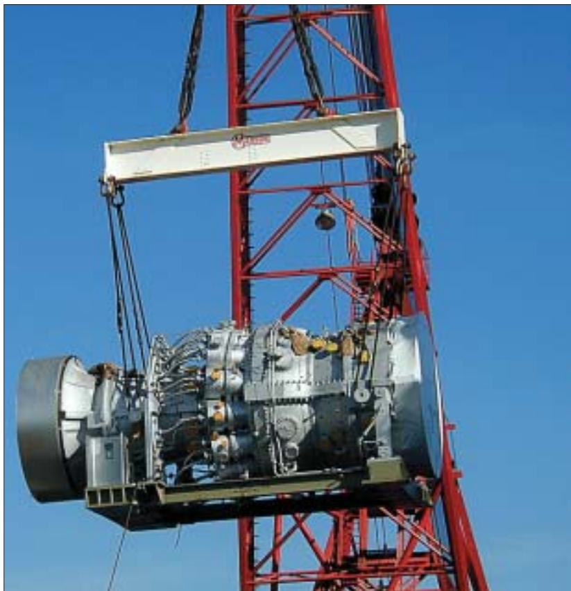
A Manson floating crane lifts a 200-ton jet engine at the Stevedoring Services of America terminal in Tacoma.
