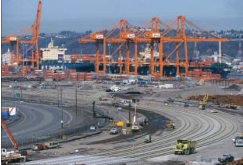
Washington United Terminals' 20 acre expansion project in progress. The expansion increased total terminal acreage (including rail) to more than 110 acres and increased on-dock rail capacity by 46%.
