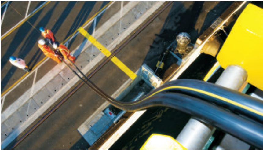
ITS plugs a ship into shoreside power at the Port of Long Beach.
